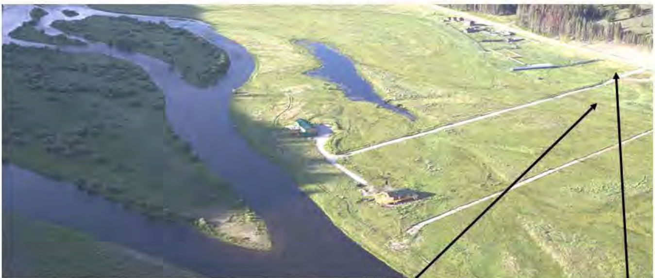
Figure II. Two manufactured homes located on the Big Hole River in Beaverhead County near Wise River. These homes are located approximately 155 feet from the river, within the 100-year floodplain, but beyond the minimum setback established by the Big Hole River Ordinance. Photo by Chris Boyer, Kestrel Aerial Services.
